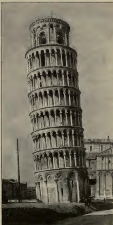
FIG. 13. The Leaning Tower of Pisa.
